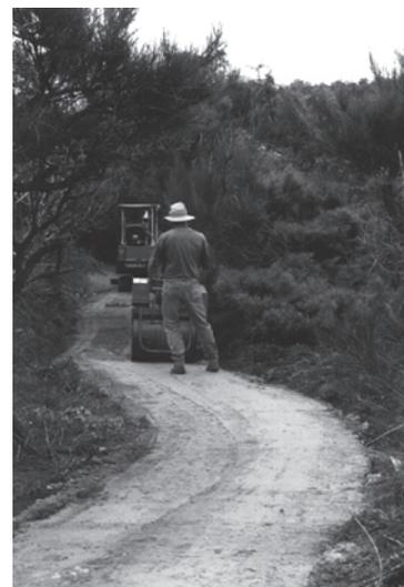
*The process for constructing the Dustex-stabilised trails at Meelup involved mixing the surfacing material off-site, transporting it onto the trail alignment, spreading it with a mini-excavator and then compacting it. The result was a very hard, smooth, long lasting trail surface suitable for a multitude of users.*
